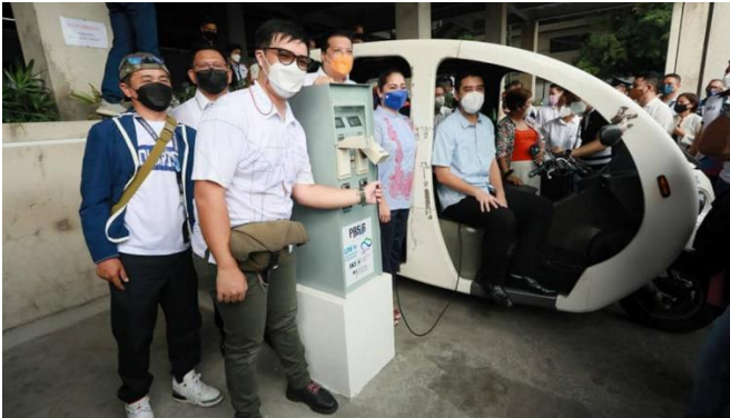
Figure 7. EVCS at Pasig City Hall Complex. 31
